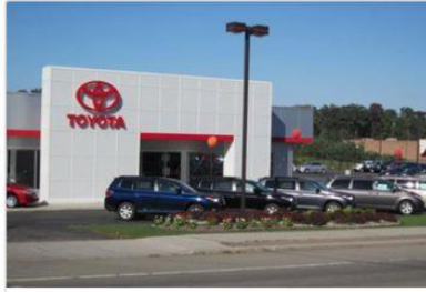
Toyota Dealership Lakewood, New York Cost Segregation Benefit ~ $87K
